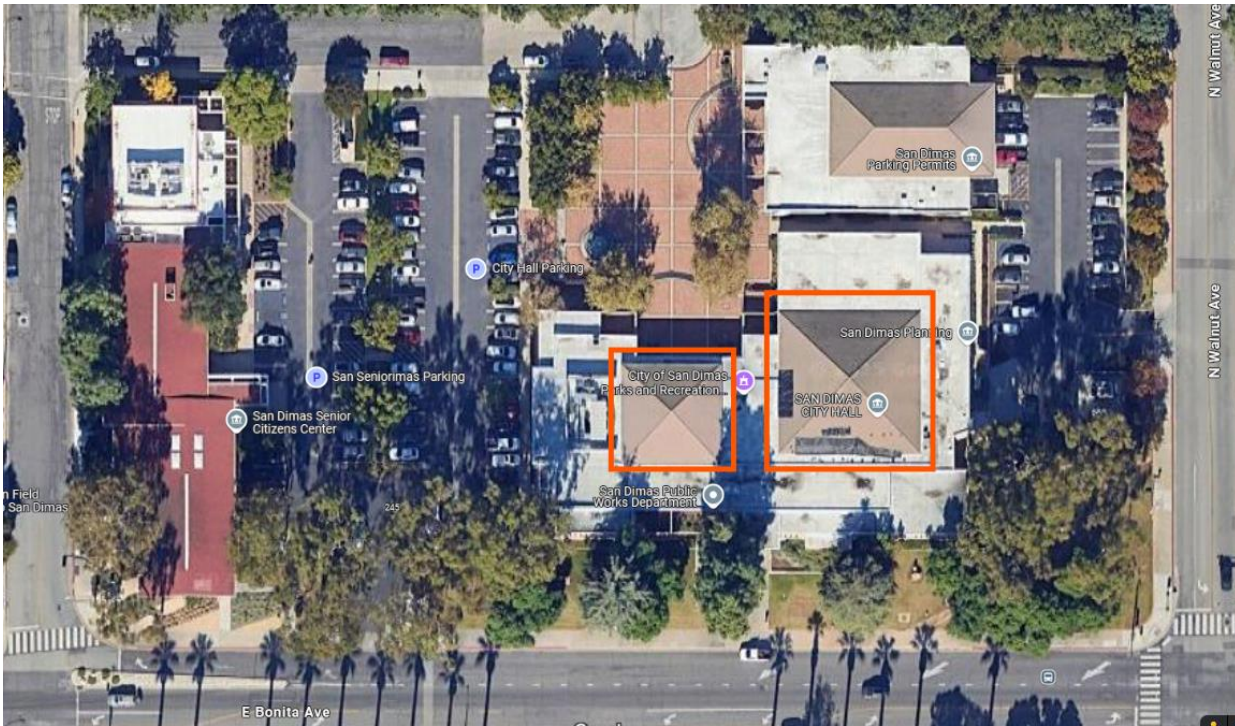
City Hall Pitched Roofs, West Roof and East Roof
